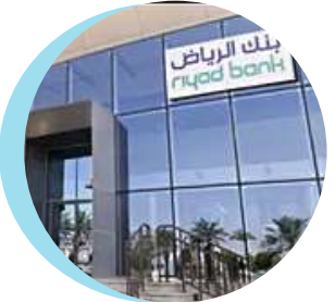
Riyadh Bank Data Center
